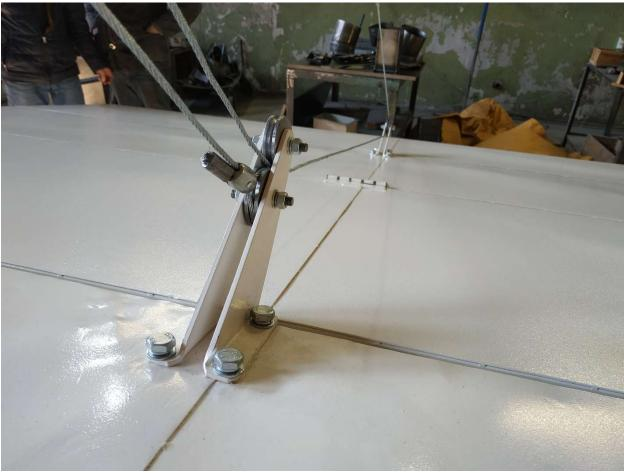
4. Installation of the unloading head of the bunker
